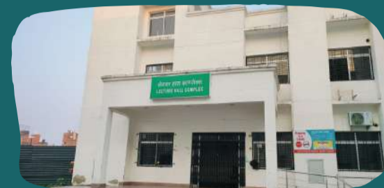
Lecture Hall Complex
